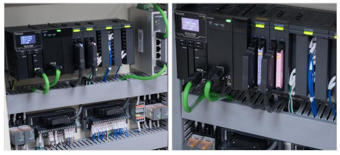
1. Keyence KV7500 PLC+Keyence module high-end bus control system, ensure the stability and extensibility of the system.
